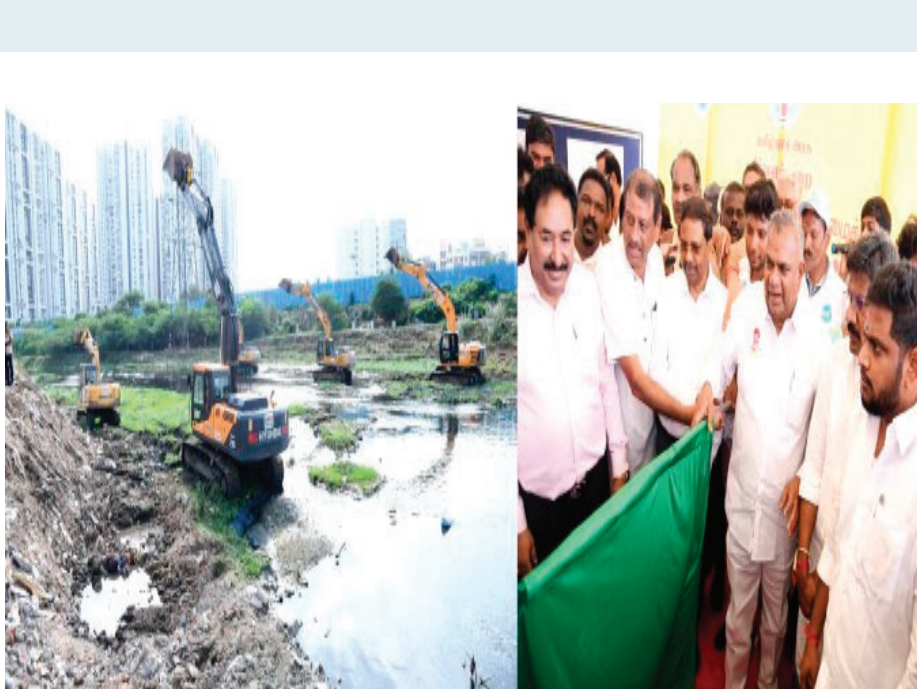
As per the instructions of the Honble Chief Minister, the Honble Minister for Rural Development and Water Resources inaugurated and inspected the desilting and restoration works of the Cooum River near Padikuppam in Aminjikarai and Okkiyam Maduvu at Okkiyam Thoraipakkam, Chennai...
