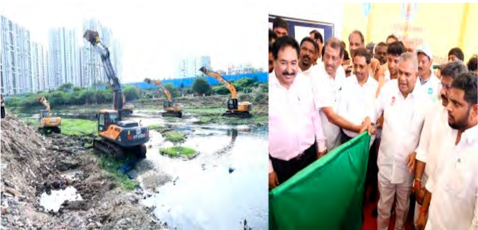
As per the instructions of the Honble Chief Minister, the Honble Minister for Rural Development and Water Resources inaugurated and inspected the desilting and restoration works of the Cooum River near Padikuppam in Aminjikarai and Okkiyam Maduvu at Okkiyam Thoraipakkam, Chennai...
