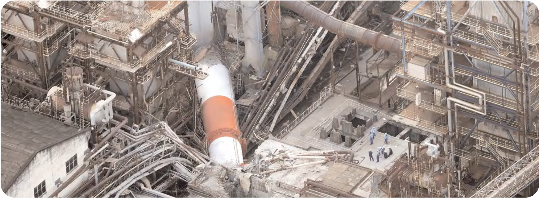
■ People trapped in Japanese mall hit by earthquake, with others missing after factory chimney collapse
