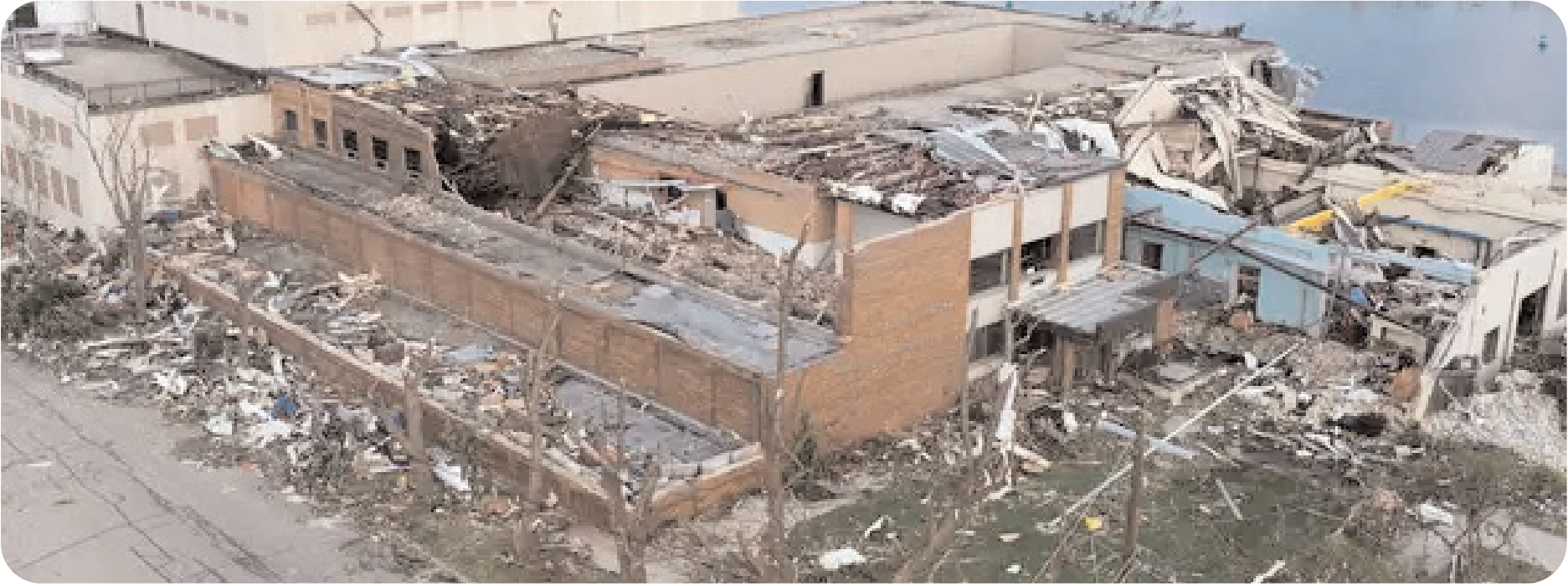
■ New storms threaten catastrophic flood zone in Indiana and could create more floods across the Midwest
