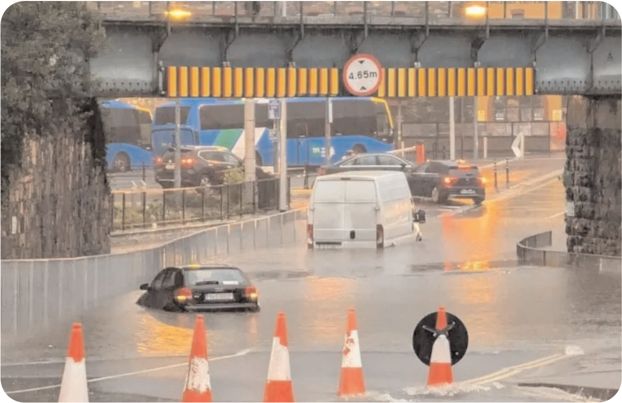
Damage being assessed after 'significant' Killarney flash floods
